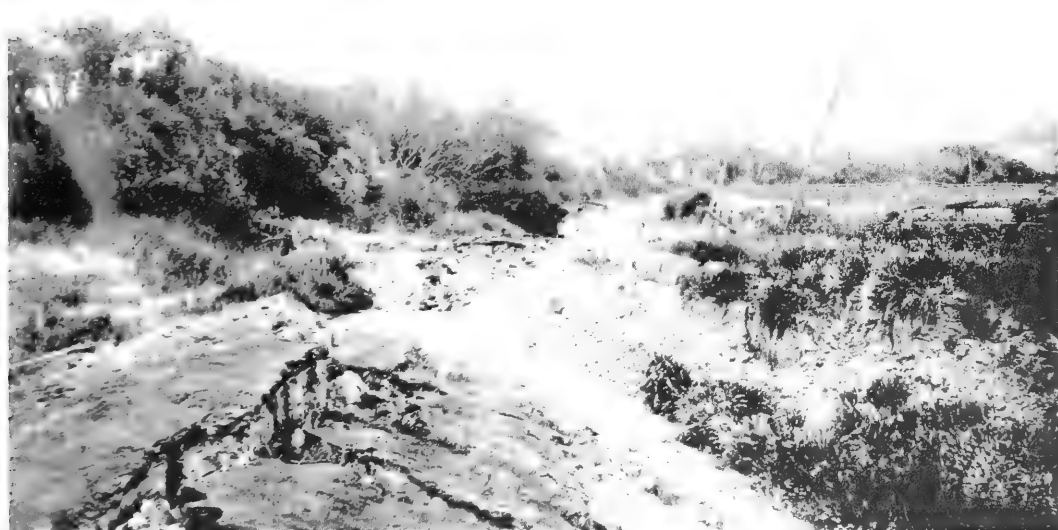
FIGURE 12. Road bed between Olema and Inverness. Road bed probably destroyed by shaking of soft ground beneath. Photograph by G.K. Gilbert. (G.K. Gilbert Collection [N-7583-F], California Academy of Sciences Archives.)
